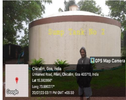
Sump Tank-II (Capacity: 4.5 L Liter)
