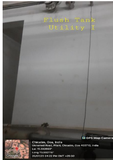
Flush Tank Utility-I
