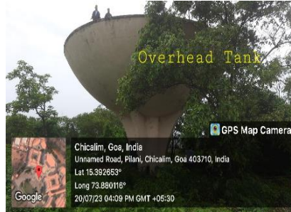
Overhead Tank (Capacity: 1.5 L Liter)
