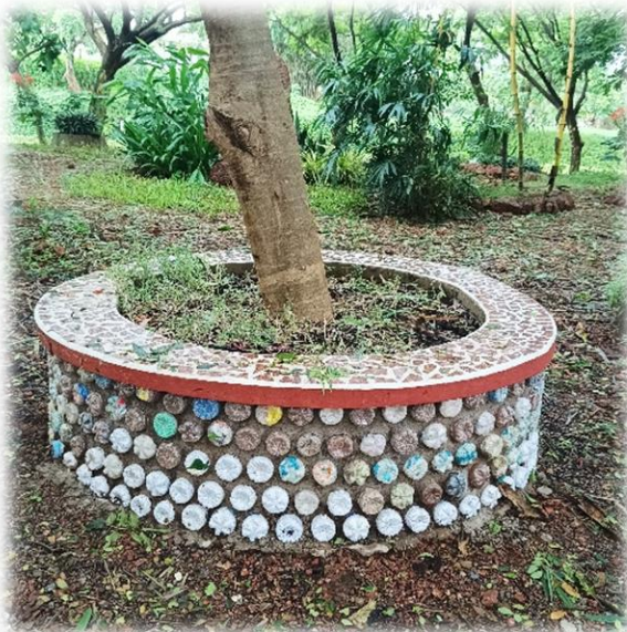
Circle planter made of eco bricks and construction remains
