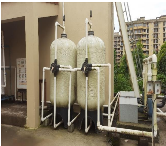
Sand and activated charcoal Filter No. 1
