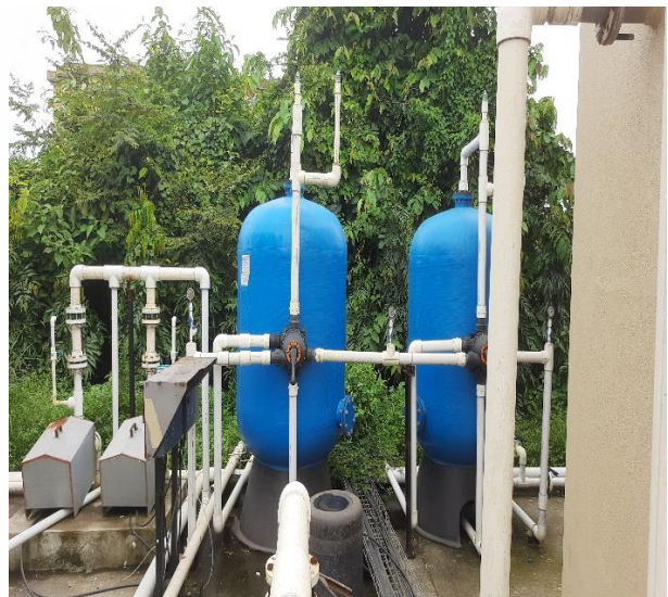
Sand and activated charcoal Filter No. 2
