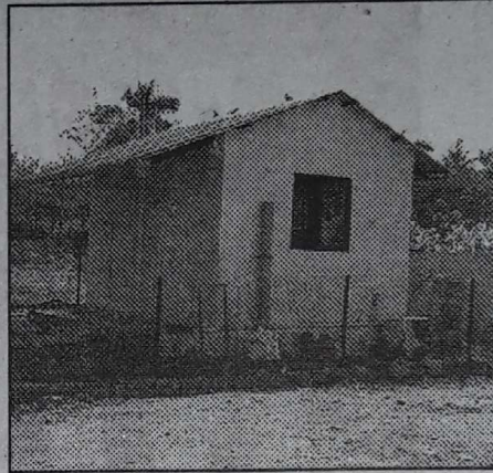
The waste treatment facility at BITS Pilani
